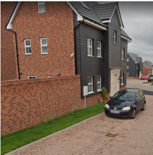
Area allocated as footway space is used for parking. The property's allocated parking is at the side of the house, which is further from the front door. The design doesn't make it clear if this area is intended to be used as parking or footway.
