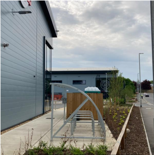
Cycle parking at a commercial building. Whilst the provision of a shelter with Sheffield stands is ok, there is no additional layer of security. The location is not overlooked by the building it serves and the proximity to the road leaves bikes vulnerable to theft.
