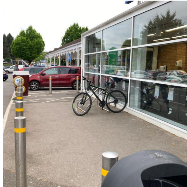
Short-term parking outside a supermarket, which partially blocks the pedestrian route in and out of the entrance and exit.
