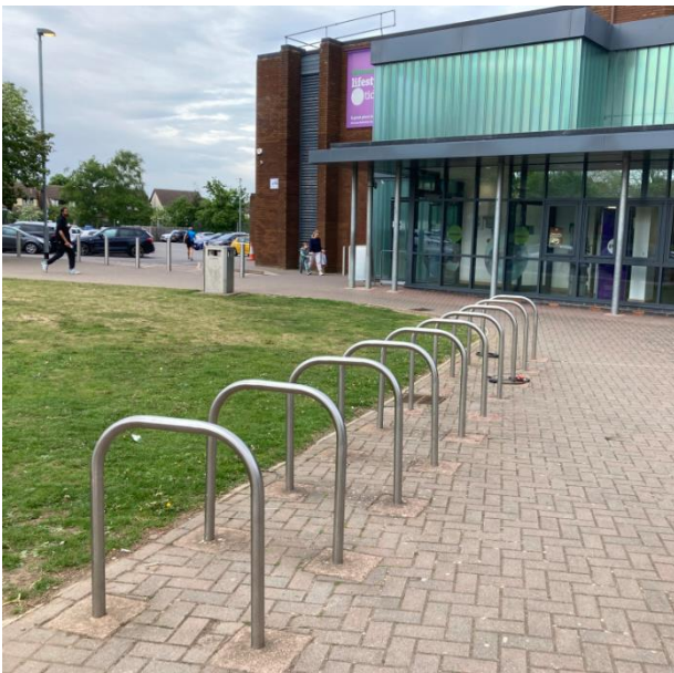
Cycle parking outside a leisure centre where Sheffield stands have been installed too close to the edge of the block paved area, meaning that bikes locked here would be partly on the grass.
