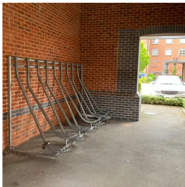
Cycle parking racks for long-term parking at residential flats. Whilst the area is covered, there is no natural surveillance of the area, and no way for residents to double lock their bikes, leaving them vulnerable to theft. The style of stand requires a certain amount of upper body strength, therefore making this style not suitable for all to use.
