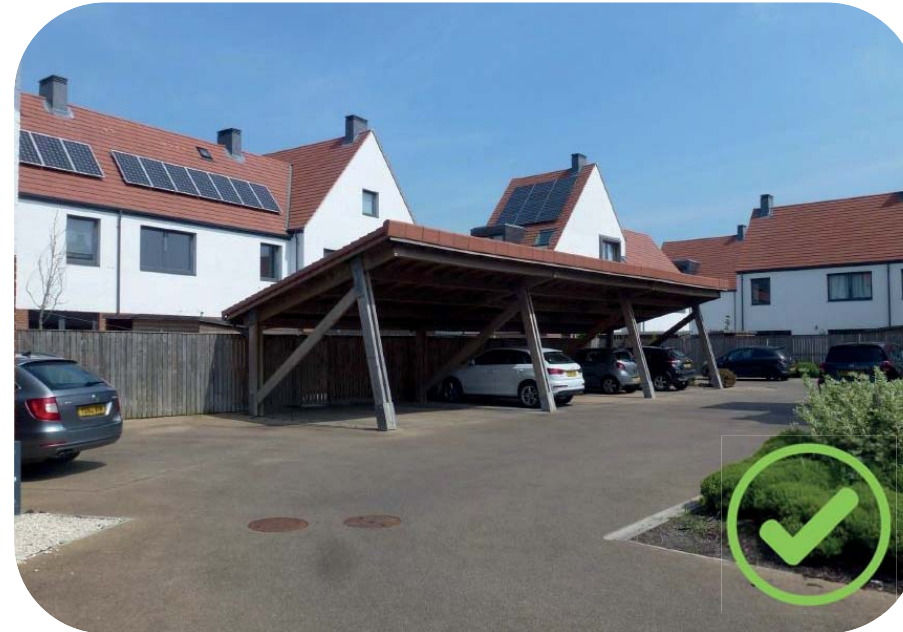
Car Barn with Possibility for Solar Panels / Green Roof (image courtesy of the Duchy of Cornwall)
