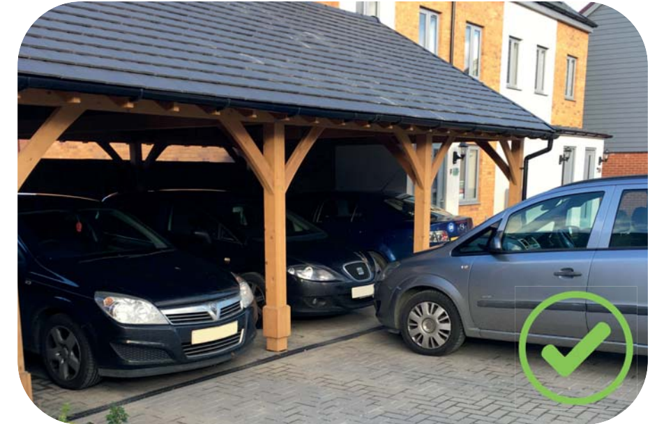
Tandem car barn, Power Station Road, Halfway
