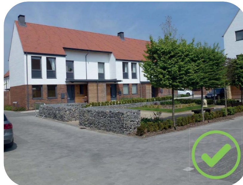
Courtyard Parking (image courtesy of the Duchy of Cornwall)
