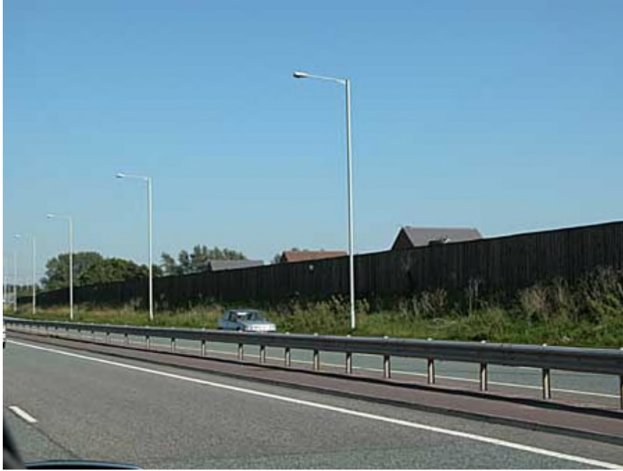
Figure MC1 Example of noise fencing
