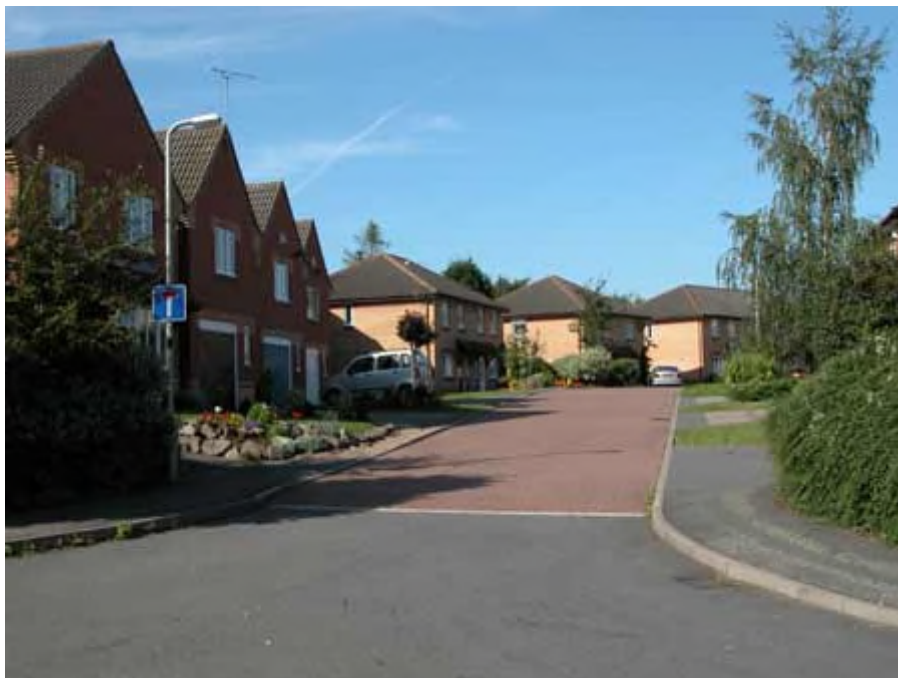
Figure GL1 Example of an entry ramp
