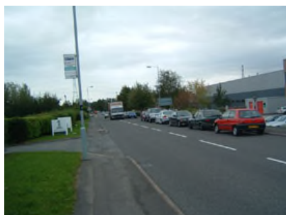
Parking causing vehicles to cross on to wrong side of the road
