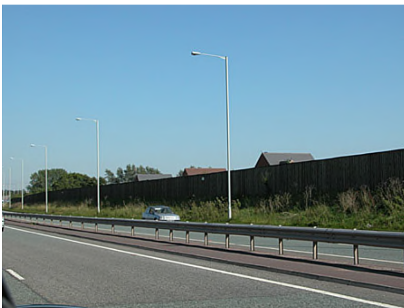
Figure MC6 Example of noise fencing
