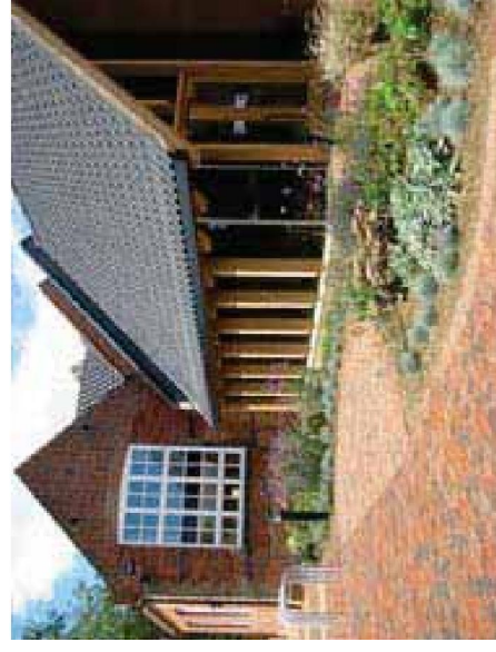
The Pennoyer Centre, Pulham St Mary: Example of retention and positive extension of an existing building
