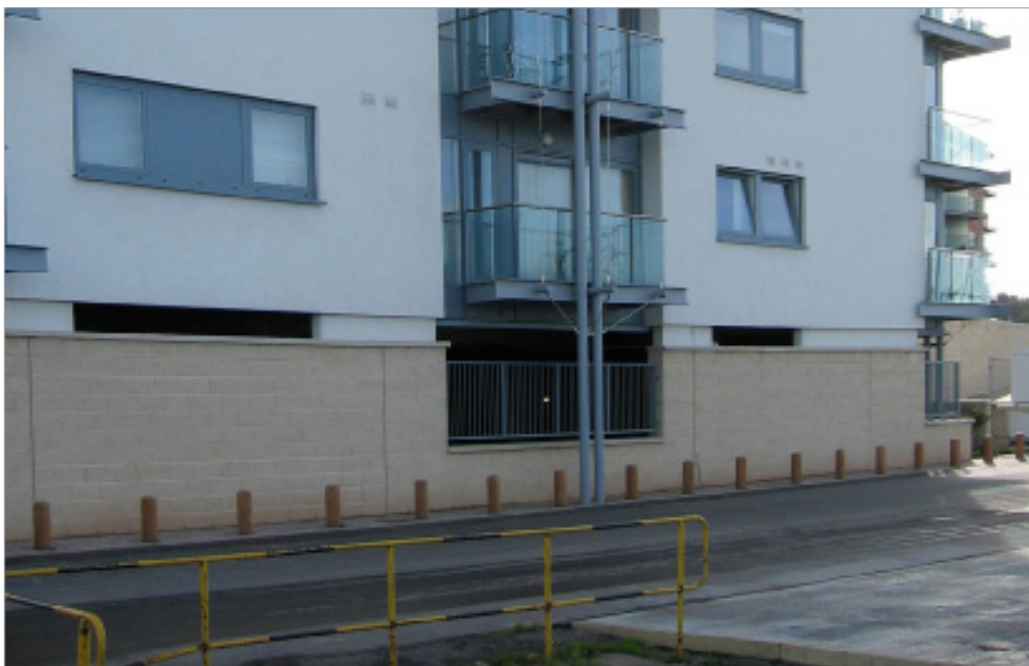
Poorly designed under-croft parking creates dead fronts and divorces the building from activities on the street
