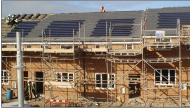
Installation of solar panels during construction phase
