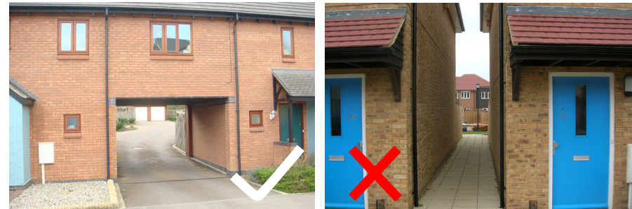
"Bridge over unit" makes a clearer definition that the rear court is private
