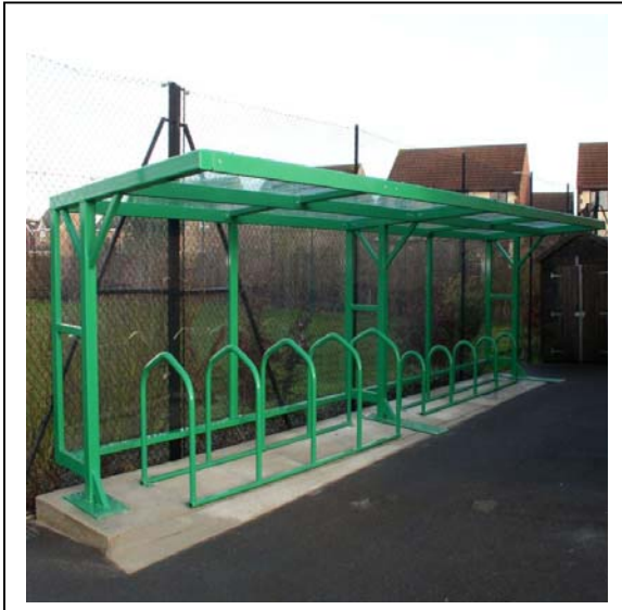
School cycle facilities with different sized "Sheffield" racks
